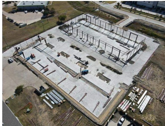
Current Aerial View
